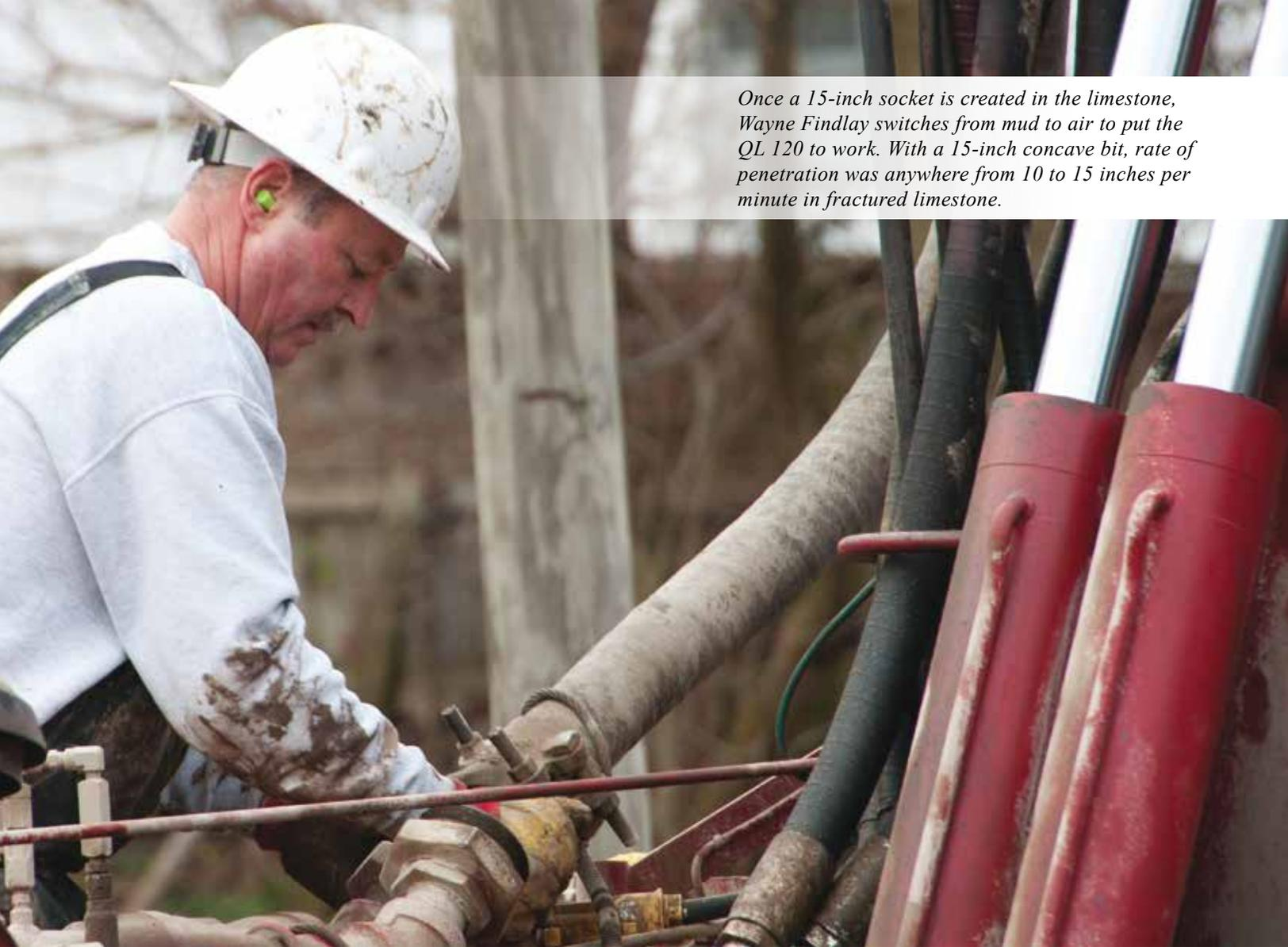
*Once a 15-inch socket is created in the limestone, Wayne Findlay switches from mud to air to put the QL 120 to work. With a 15-inch concave bit, rate of penetration was anywhere from 10 to 15 inches per minute in fractured limestone.*
