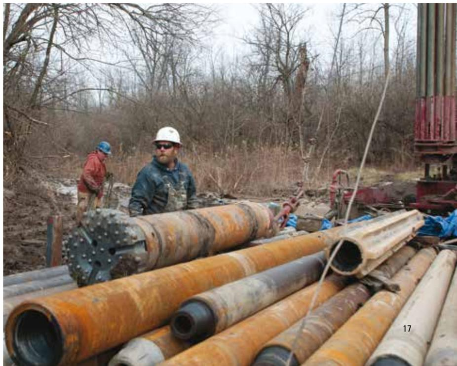
» Findlay cleaned the cased top portion of the well and sent down a stepped tri-cone starter bit into the limestone. This was an 18-inch diameter reamer of bit thirds with a 15-inch tri-cone extending ahead of it. The pilot bit created a perfectly centered rock socket to start the QL 120 with a 15-inch bit.
